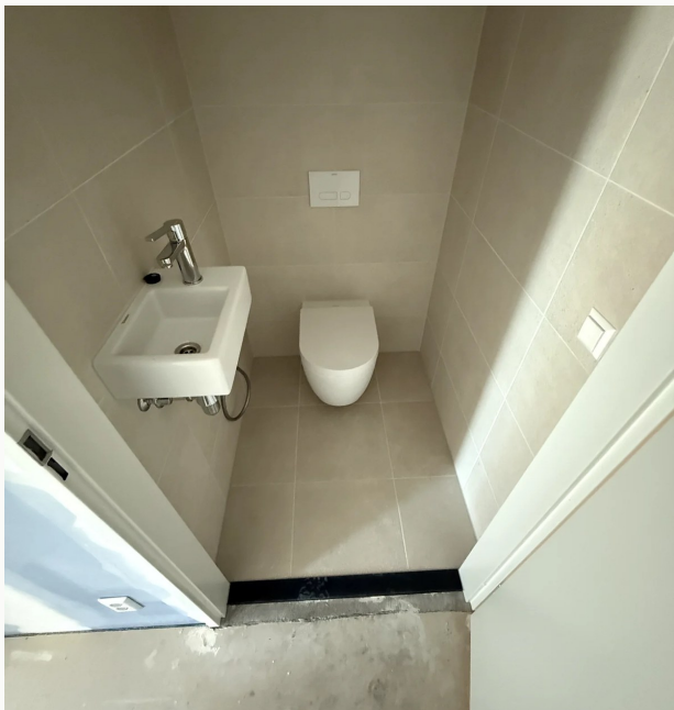
Separate toilet — completed finish, independent from the bathroom
